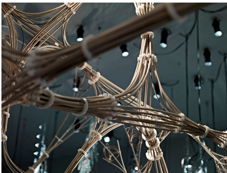
Figure 4.1: Detail of demonstrator “The Rise” in Paris, showing rattan bundles managed by HDPE “packing nodes” and the rattan deployed in oppositional active-bending branching moment connections as organized by HDPE “stars”. Photo by Anders Ingvartsen
